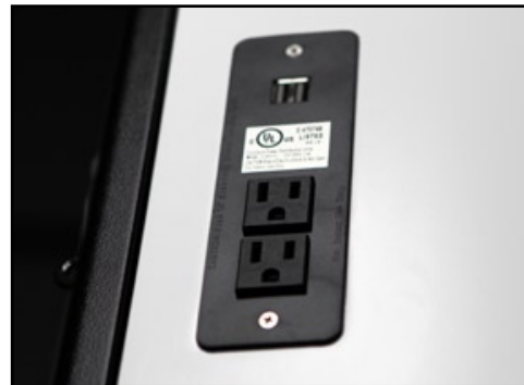
External Power Outlets
