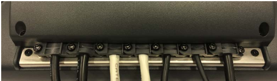
Fig. 8.11: Cable cover closed and screwed together
