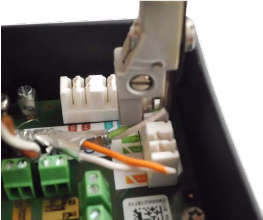
Fig. 63: Network wires connected using LSA+/Krone tool
