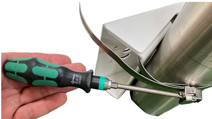
Fig. 42: Tighten the straps
