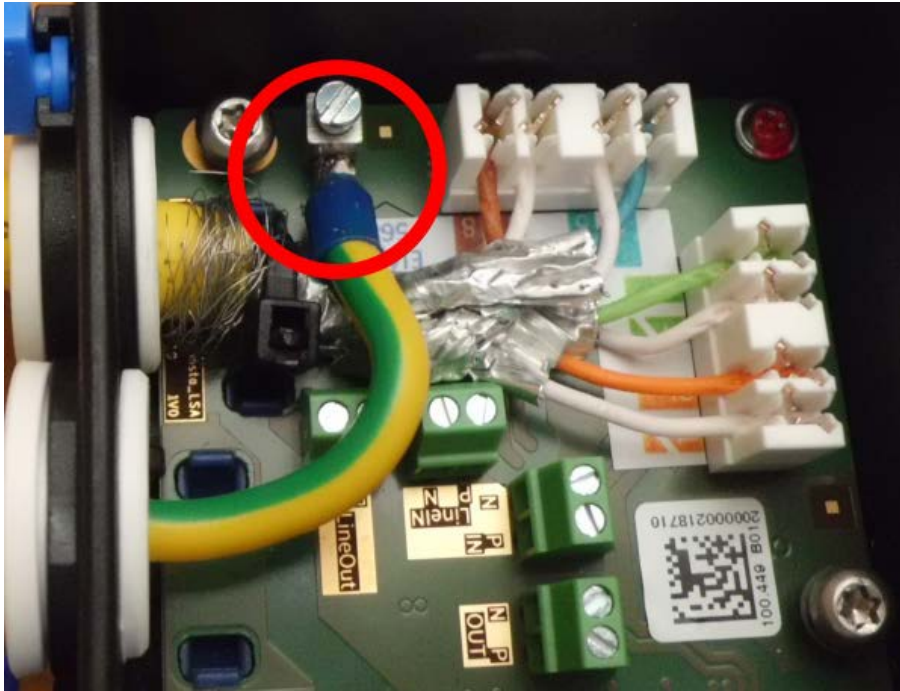
Fig. 66: Ground wire connected to terminal
