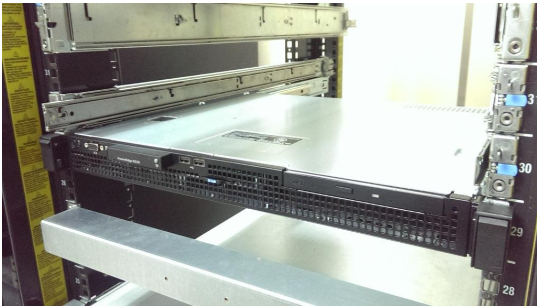
Figure 7. R220 mounted in a 4-post square hole rack
