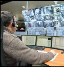
Command and Control Rooms
