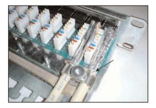
3b. If the STP cable has an outer diameter of more than 0.2" (6 mm), bend back the copper braid and place the braid under the bracket. (Place the bracket exactly where the braid bends.)
