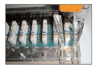
5. Arrange the wires according to the color. Use a punchdown tool to terminate each pair.
