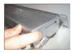
9. Insert the front side of the cover into the panel hood.
